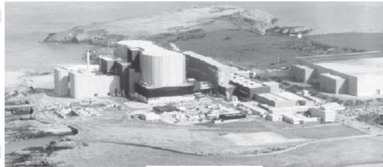
Power station project.
