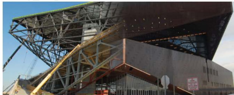
CONSTRUCTION SITE PROGRESS PHOTOGRAPHY
