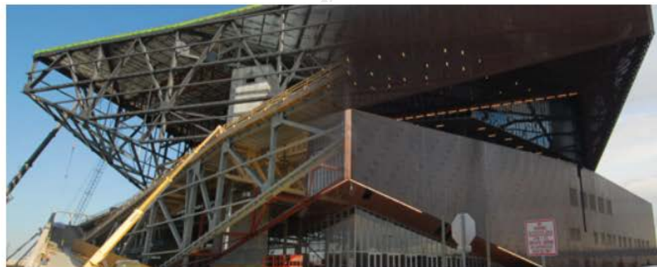
CONSTRUCTION SITE PROGRESS PHOTOGRAPHY
