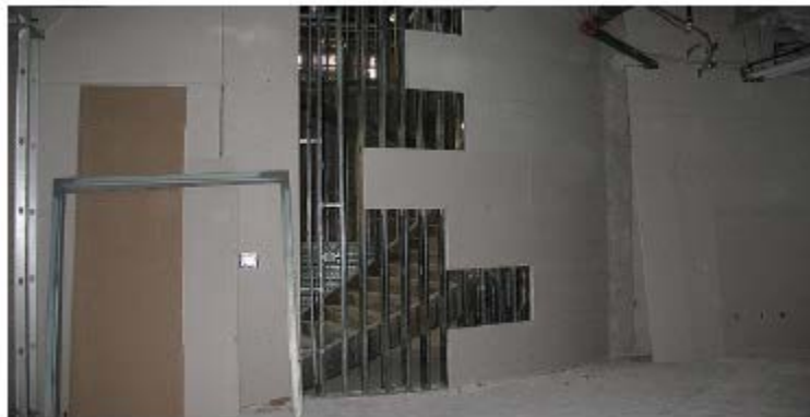
Drywall installed before conduit
