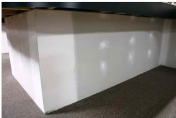
Carpet installed before paint
