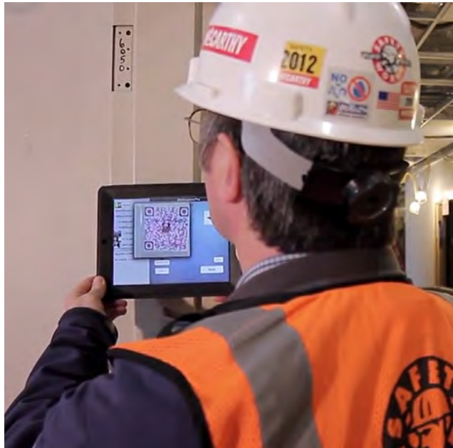
Figure 6.37 Superintendent using BIM Anywhere to scan QR codes for quality control in the field
