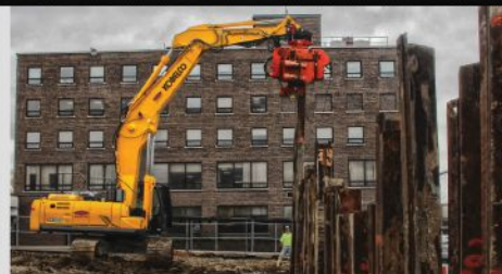
V-2 Esc Vibratory Pile Driver • 25 Tons of Driving Force
