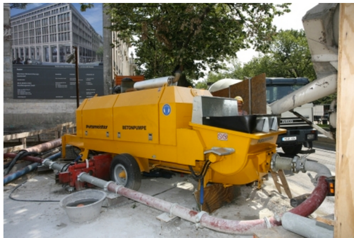
FIGURE 8- Example of a Stationary Concrete Pump connected to a pipeline
