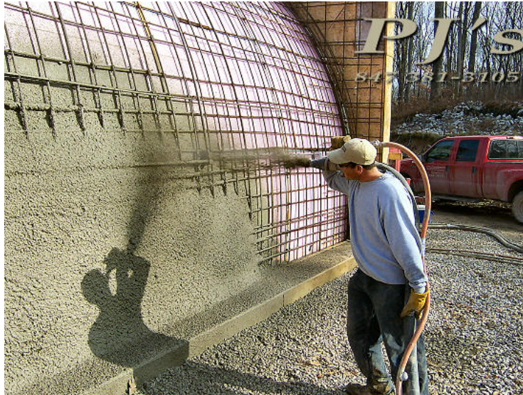
FIGURE 17- Example of a Nozzle attachment spraying concrete
