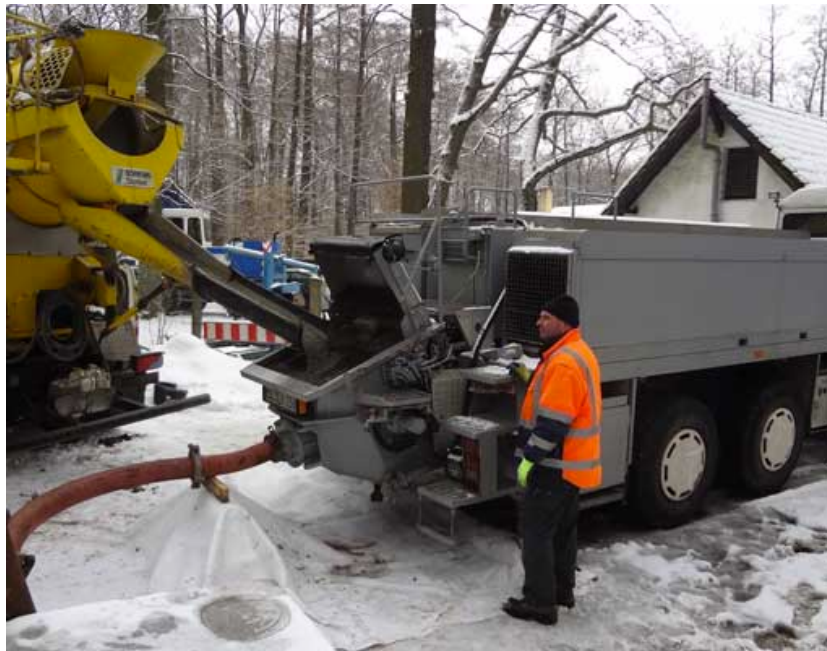
FIGURE 11- Example of Pump and Separate Pipeline configuration being supplied by a Concrete Mixer Truck
