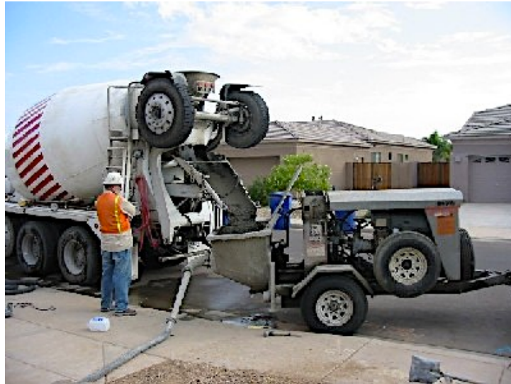
FIGURE 9- Example of a Trailer Pump attached to a Concrete Mixer Truck
