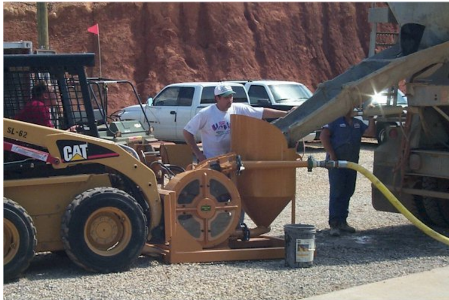
FIGURE 6-Example of a functioning Peristaltic Concrete Pump
