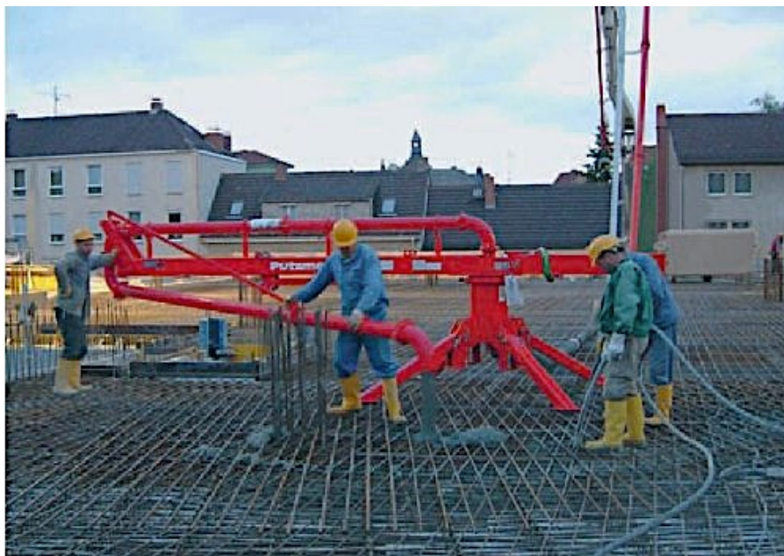
FIGURE 16- Example of a Distribution Boom being used to facilitate the pouring of concrete.
