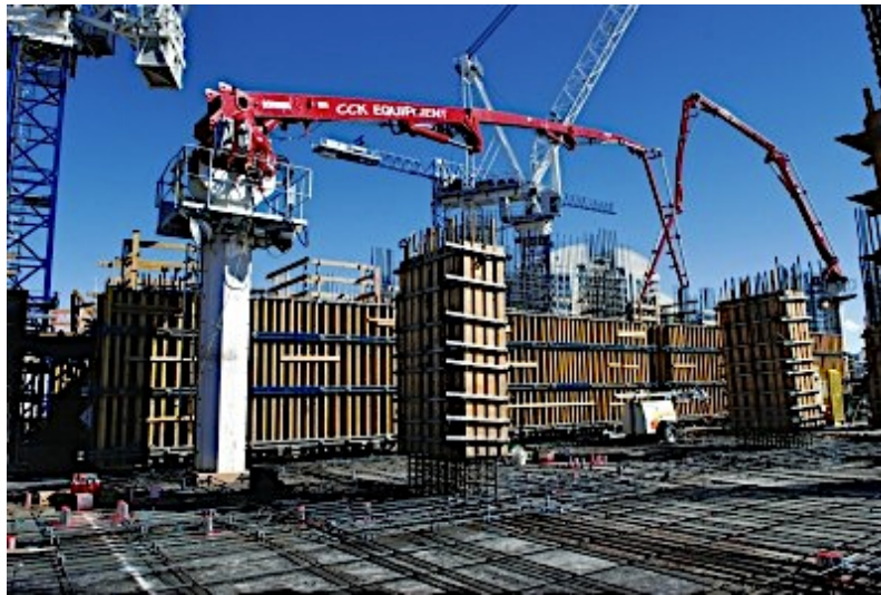
FIGURE 14- A construction project using several Tower-Mounted Booms for concrete pouring.
