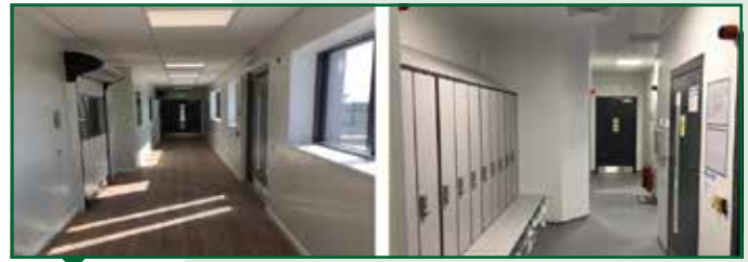
Figure 4. Module Internal Finishes – completed off-site
