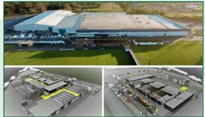
Figure 1. Modubuild Off-Site Fabrication Facility
