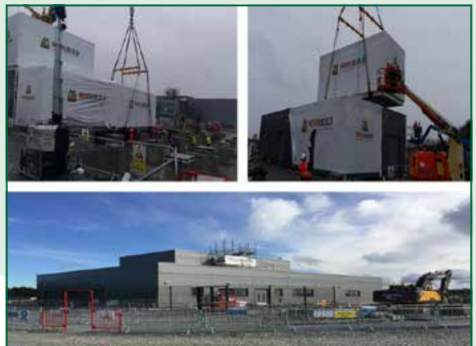
Figure 3. On-Site Module Installation, & Assembled Building
