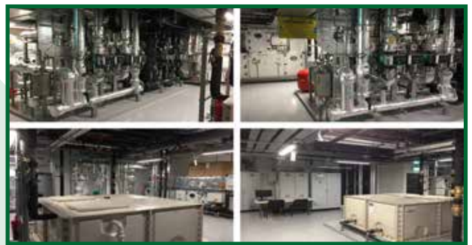
Figure 5. Plant Room & FAT Testing Station completed off-site
